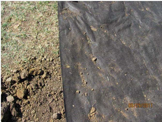
This is a close up of the geotextile used. Recommend extending it at least 8 feet beyond the outside of the tire and covering with gravel
