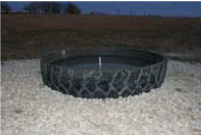
Tire with water filled to cover concrete for curing. Let this cure for 3 weeks.
