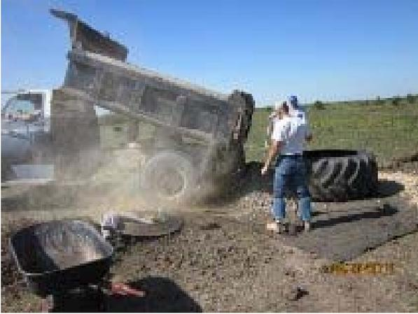
Coarse gravel is placed around tire tank over geotextile fabric.
