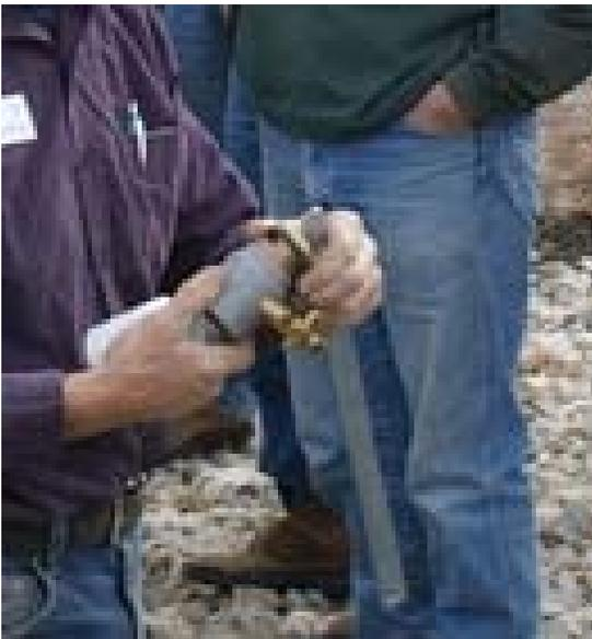
Showing the valve with a winter minimum continuous flow valve installed.
