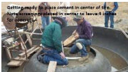
Inside of tire is filled with sand or lime screenings and tamped to allow 4 to 6 inches of concrete depth.
