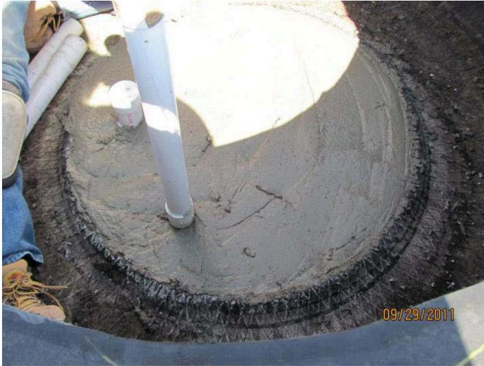
Concrete is poured to desired level and ready for final troweling. Note relation of concrete to the tire bead and the joints on the inlet and overflow pipes.
