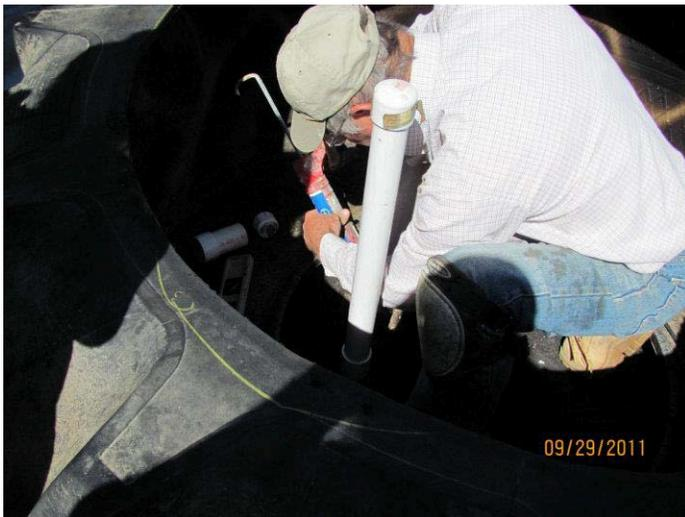
Sealing with silicone around the inlet and outlet pipes helps to prevent leaks.
