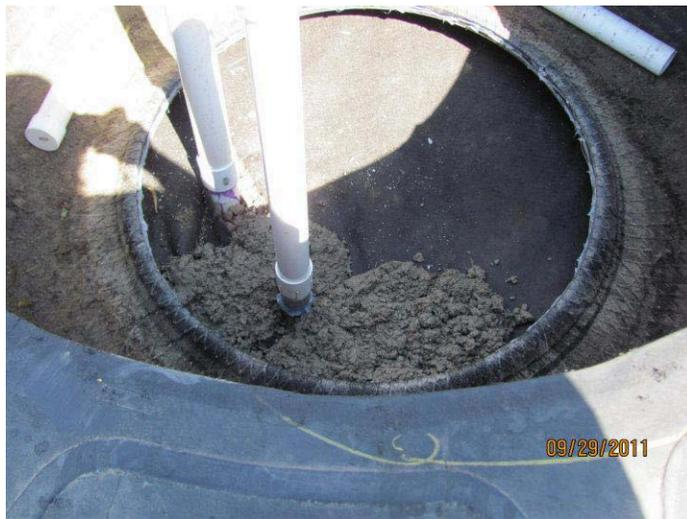
Beginning to place concrete mix. Make sure it is not too stiff to allow working it under the rim.
