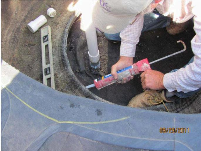
A heavy bead of silicone helps seal the concrete to the tire rim.
