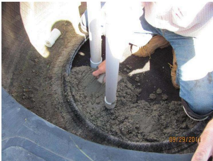
Working the concrete mix under the rim to ensure good contact.
