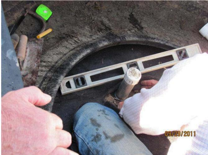
Tire is placed over geotextile and checked for level.
