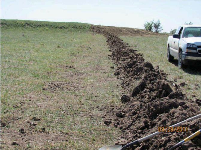
Note: Special attention should be paid to the area where the pipe goes through the dam. The trench in this area should be well compacted to ensure against seepage along the pipe. An anti-seep collar can also be used to help cut off any potential seeps.
