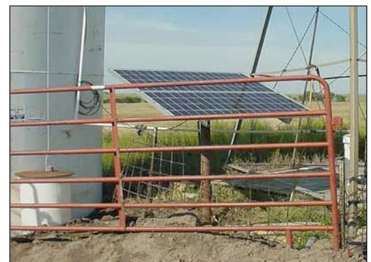
*A solar pump brings water from a pond to the storage tank at the left where it is provided in a tire tank. All above photos by H. George.*
