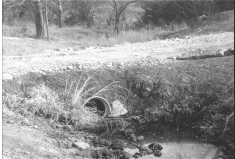
*Ken built a couple of stream crossings (right) for his cattle, using gravel over engineering fabric. The fabric (left) will help keep the gravel from sinking into the mud during wet weather, and is cheaper than concrete.*
