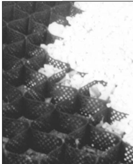
*Ken placed a freeze-proof watering tank below the fenced-off pond (above left), and installed a gravel pad around the waterer to reduce erosion and run-off in a high traffic area. He used a geosynthetic product called geo-web around the tank (above right). It is a honeycomb material filled with gravel that will hold the gravel in place and allow water to drain away.*
