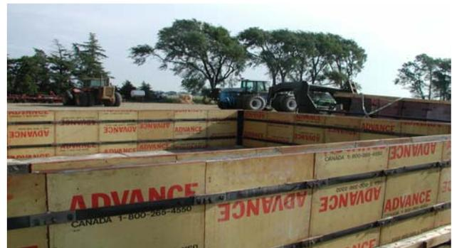
*Above photo shows the Sanders fuel containment before the cement forms are removed. The fuel containment structure is a sixteen by sixteen foot concrete structure with sidewalls tall enough to hold 110% of the fuel located there in case of a spill.*
