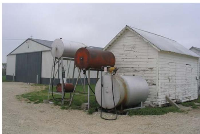
*BEFORE:* The former fuel storage system on Chris Visser’s farm included a diesel tank with a seep. After completing the RFFP environmental assessment, Chris saw the need to replace the tank and implement containment tanks.
