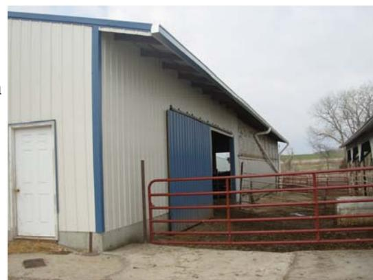
*Guttering was installed on the freestall barns and the water was directed straight to the stream behind the farm. This prevents the water from crossing the lots and becoming contaminated.*
