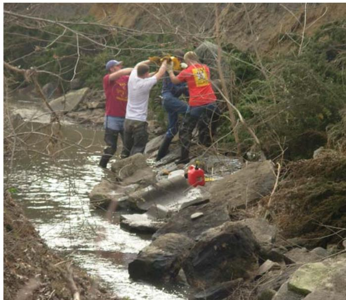
*As part of the revetment, Briane Coomes, Tyler Hamman, Joe Schmitz, Ben Davis, and Charles Barden (left to right) drive a duckbill anchor into the stream bank. The anchors will hold the cedars in place using an attached steel cable.*
