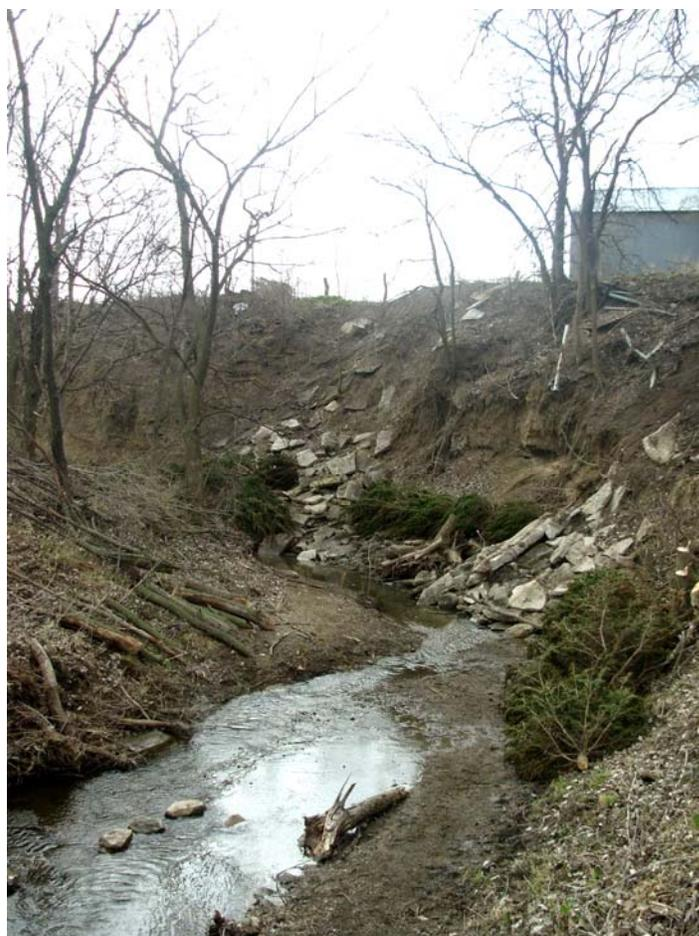
*Above is the erosion that is taking place on the Schmitz's stream. Charles Barden said he and the team moved this concrete in an attempt "to cover the "toe" or bottom of the stream-bank." "By stopping the lateral movement of the creek, the vertical slope above it can begin to revegetate." he said.*
